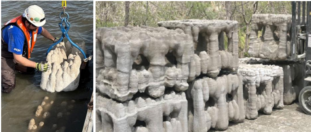
Natrx installation; Source: Natrx website
